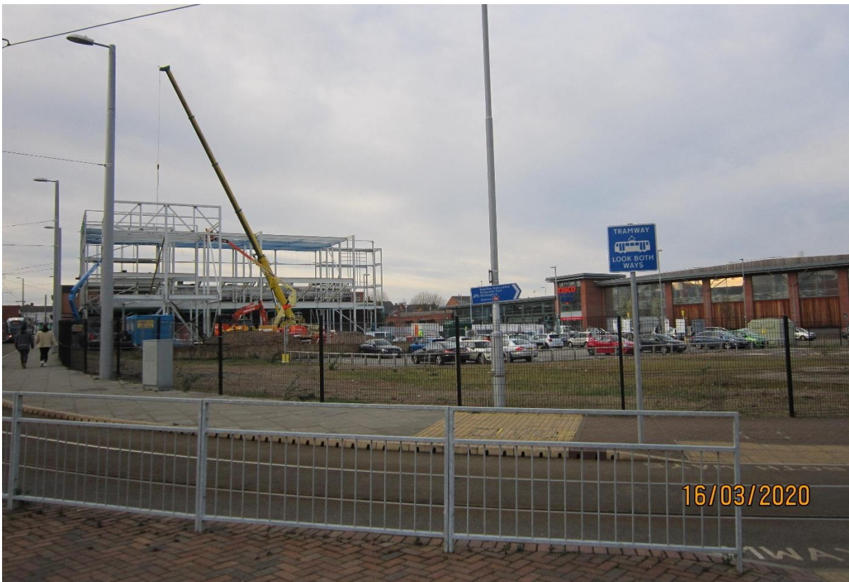
Middle Street/Styring Street corner
